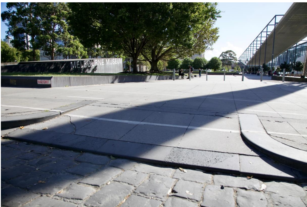
Image 4- a photo showing a 2-metre-wide driveway in the taxi zone on Nicholson St
