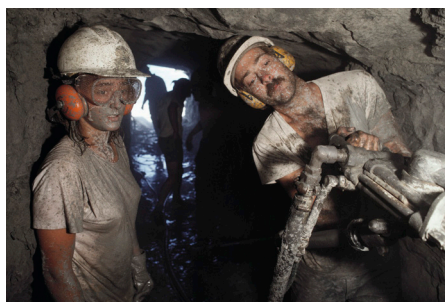
Fig. 8. John Wilson and Corrie Williams. Drillers! Here, these two long term volunteers are drilling a series of holes for explosives in a tunnel at Dinosaur Cove. Corrie's job was to hold the drill steady when John began each hole so the tip remained in the same spot on the irregular rock face. Neither of them had done anything like this previously. One of the many examples of participants learning new skills on the job for the project to succeed. (Photograph by ©Peter Menzel/ menzelphoto.com .)
